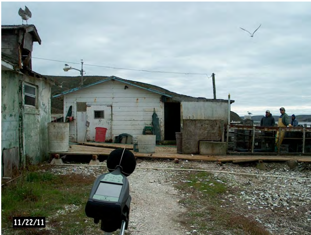
Photo 6. Building (with openings) Housing Air Compressor
