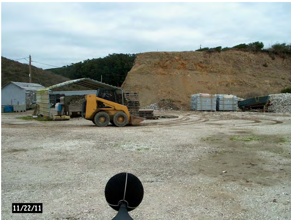
Photo 8. Frontend Loader Hauling Shells to Piles
