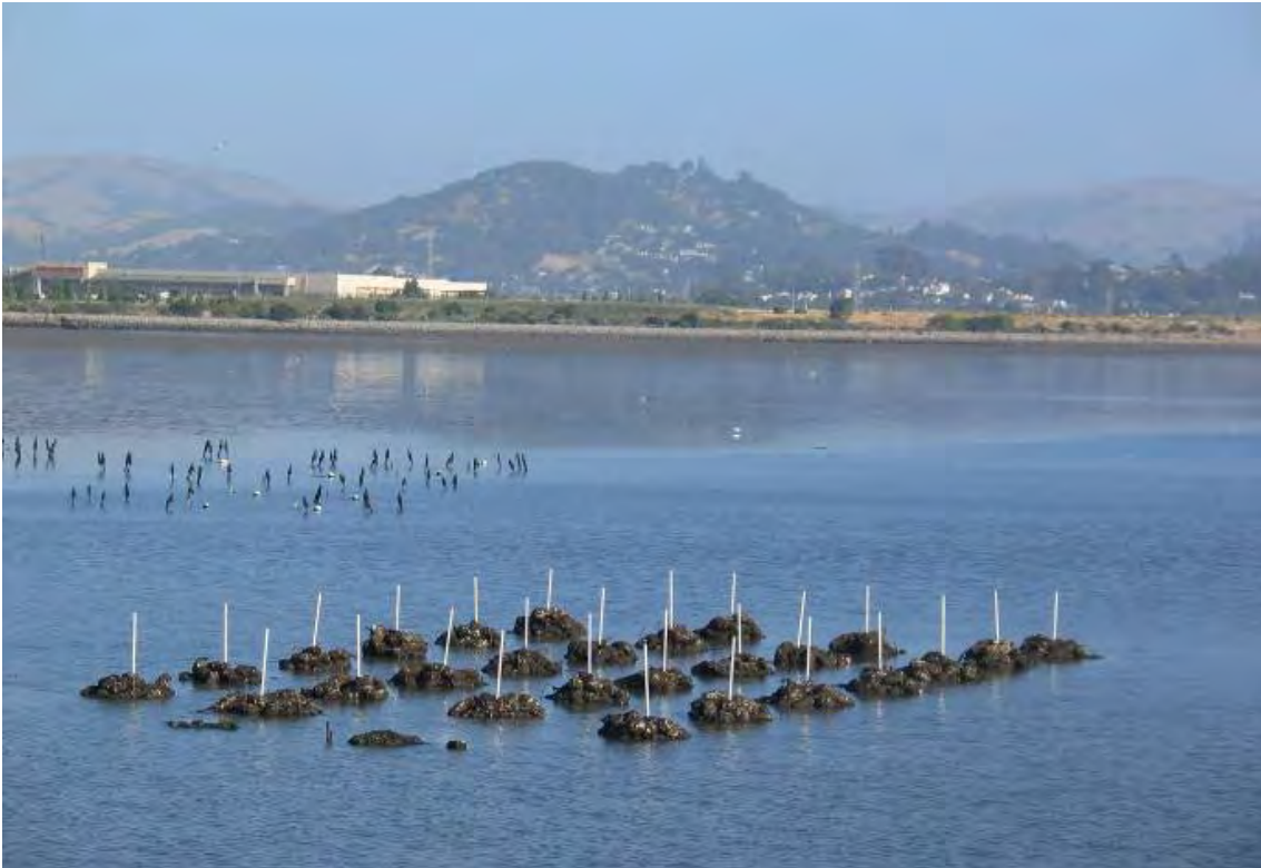
Figure D-1. A low tide view of one of the reefs constructed from oyster shells donated by Drakes Bay Oyster Company.
